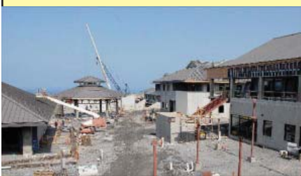
David Lyman coordinating construction of the West Hawaii Civic Center..
