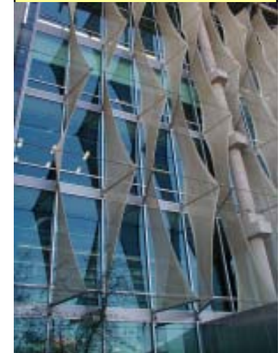
Sail-like shading devices grace the north façade of Will Bruder's Phoenix Central Library.
